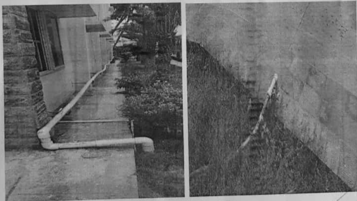
Rainwater harvesting system
