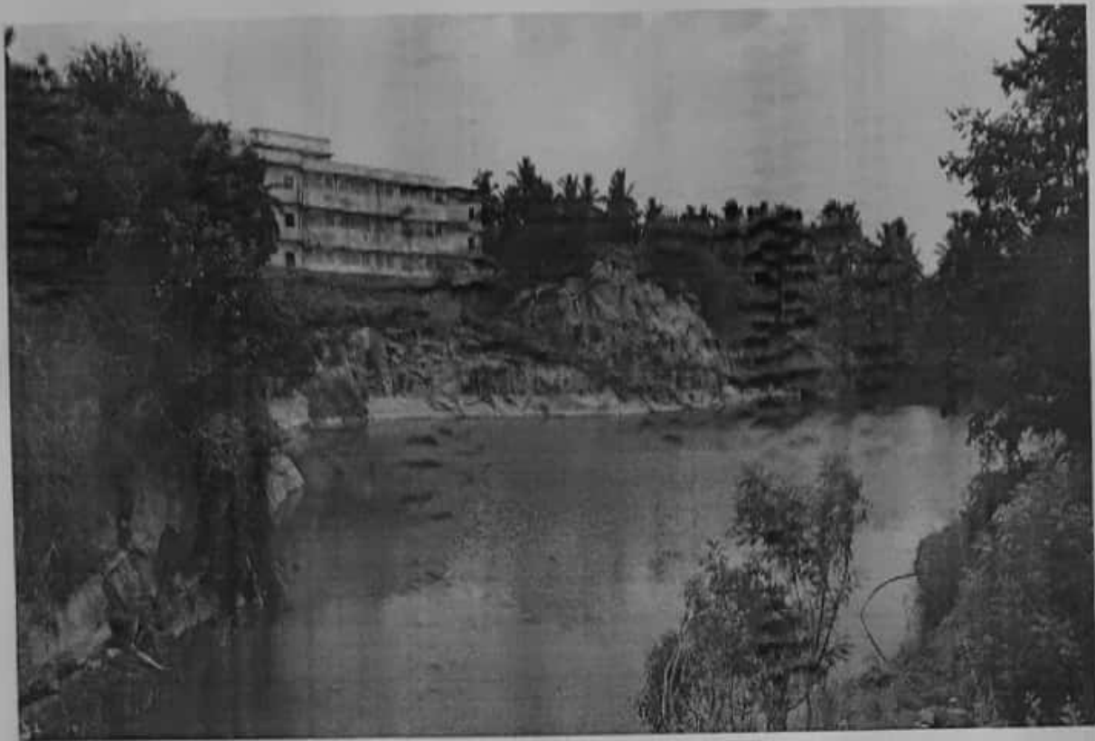
Rainwater harvesting system(POND)
